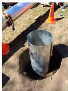
As you can see, the hole is very clean with no soil to clean up and remove from site. The base section of pole is then inserted in the hole, back filled and compacted using an appropriate fill for the surrounding soil conditions.
