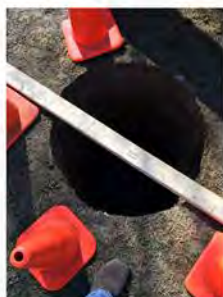
As you can see, the hole is very clean with no soil to clean up and remove from site. The base section of pole is then inserted in the hole, back filled and compacted using an appropriate fill for the surrounding soil conditions.
