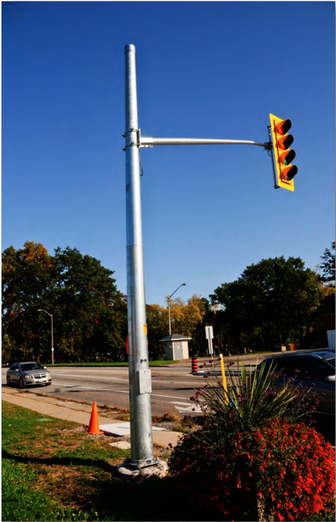
INSTALLED SECTIONAL STEEL POLE—THE SAFEST IN THE INDUSTRY
